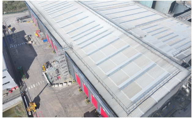
Secondary view showing perimeter gutters, adjoining roof sections and operational access constraints.
