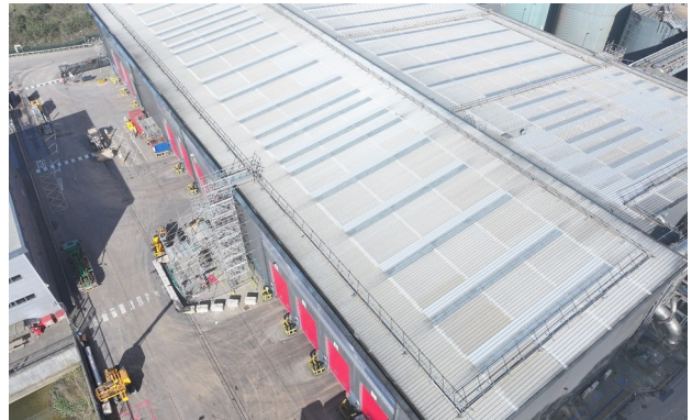
Alternative angle used to review drainage paths, rooflights and perimeter details.
