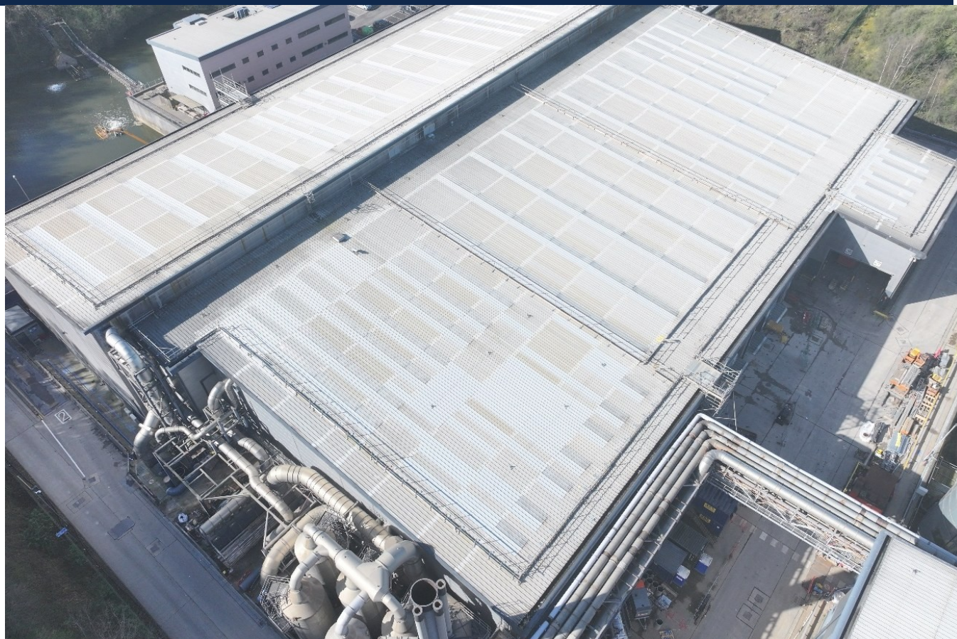
Example industrial roof viewed during an aerial inspection. Site identifiers have been removed.
