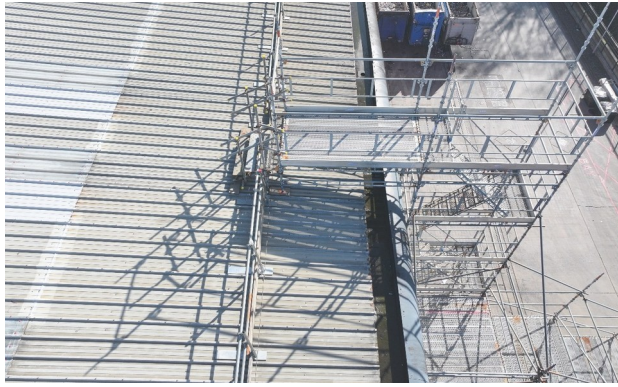
Temporary scaffold access positioned beside the roof edge.
