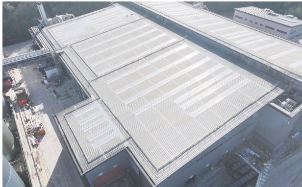
Oblique aerial overview used to establish roof form and inspection zones.
