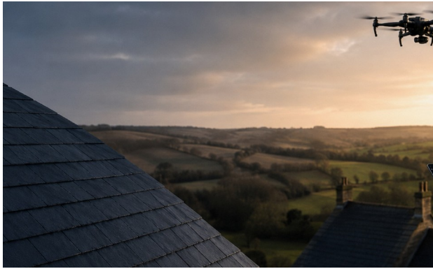
Pitched roof surfaces should not be accessed without suitable work-at-height controls.
