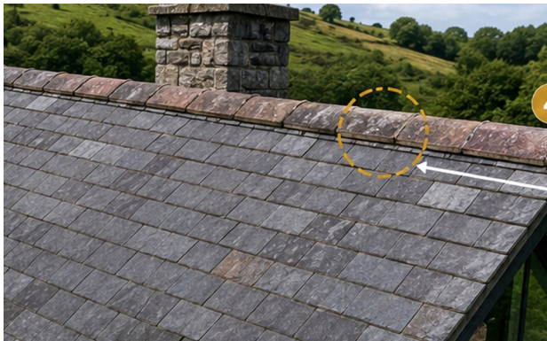
Eaves and valley junction reviewed for moss, debris and restricted drainage.
