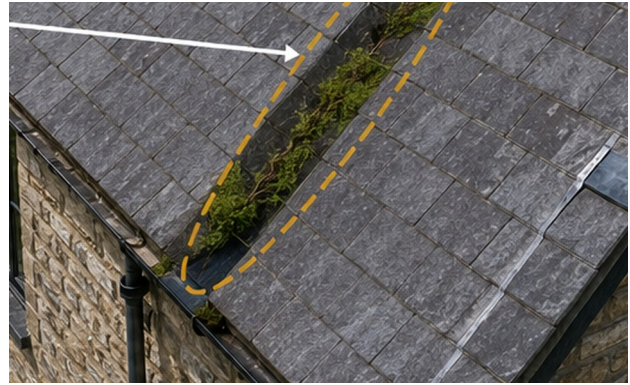
Drone-assisted review used to reduce unnecessary access onto pitched roof surfaces.
