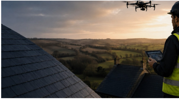
Principal slate roof slope reviewed for displacement, surface weathering and ridge condition.
