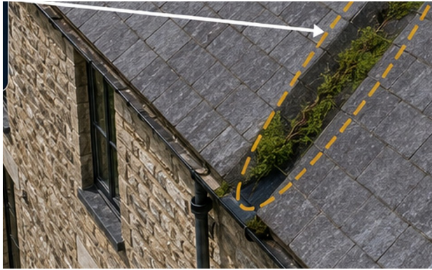
General roof slope and external junctions reviewed for visible weathering and defects.
