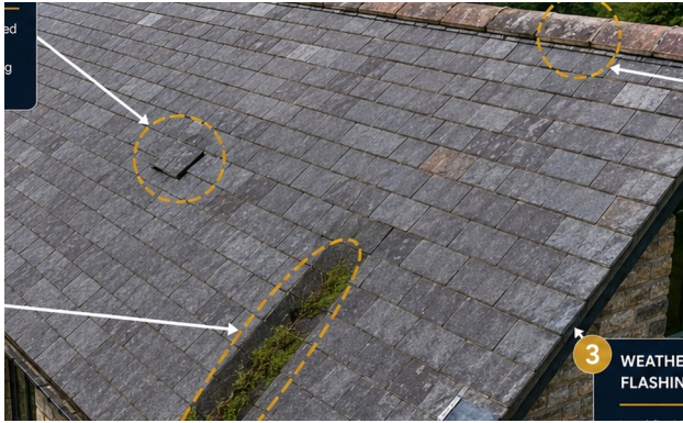
Masonry chimney and ridge details reviewed for pointing, flaunching and weathering.
