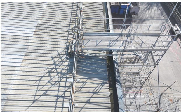
Temporary access arrangement beside a commercial roof edge.
