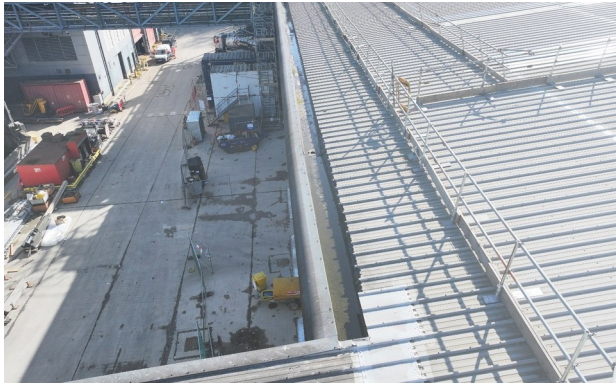
Perimeter gutter and adjoining roof junction reviewed for debris and drainage restrictions.
